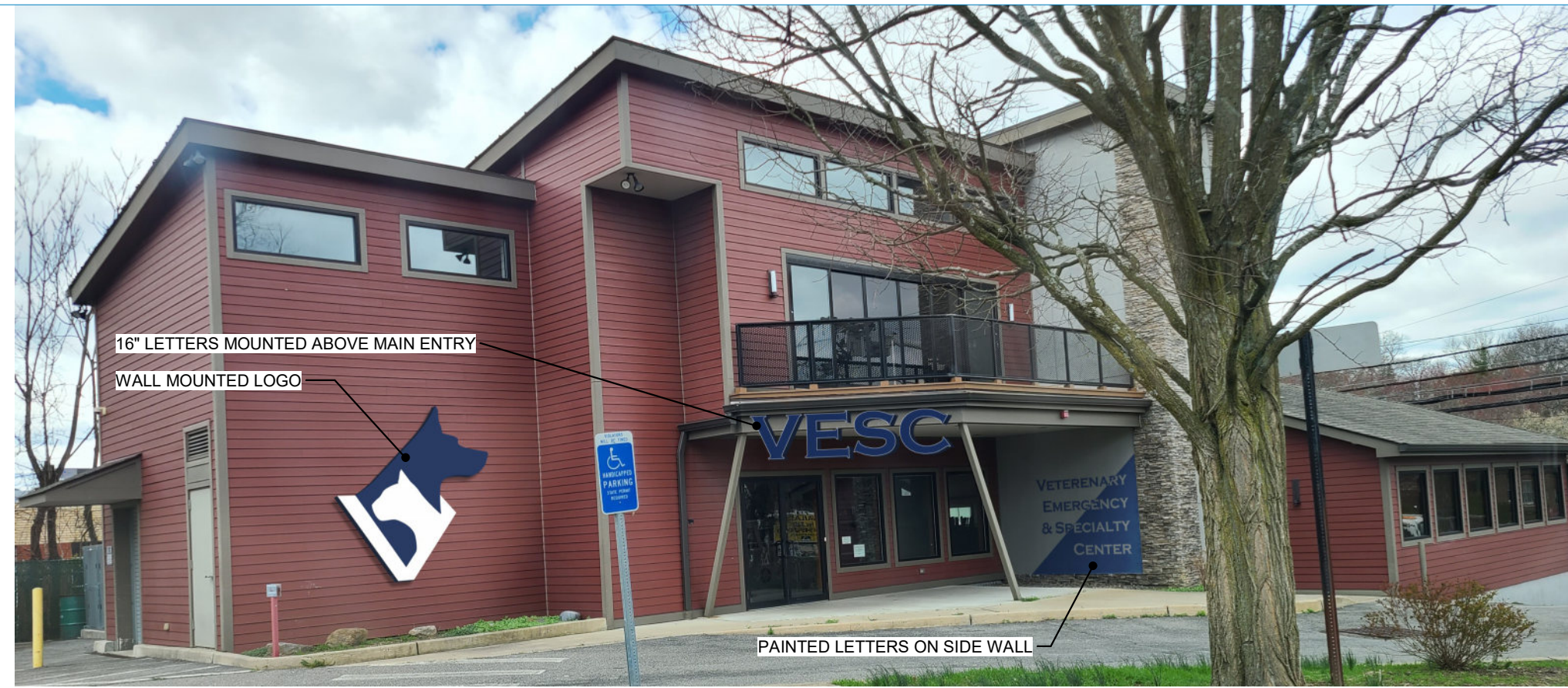
NEW SIGNAGE AT MAIN ENTRY ON EAST FACADE
